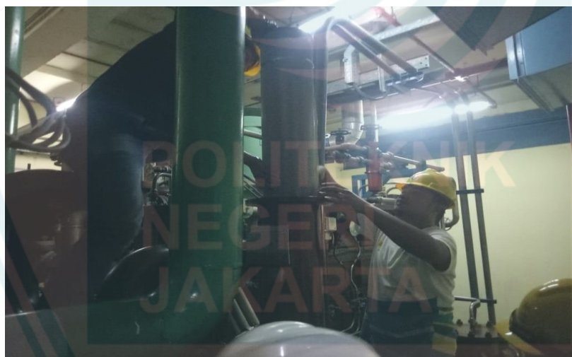
Gambar 1 Pembersihan Filter Oil
