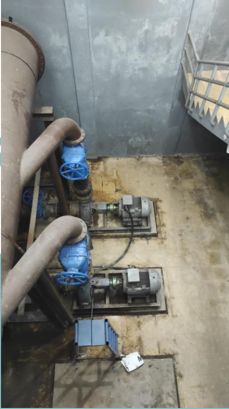
Gambar 1. Pompa Intake
