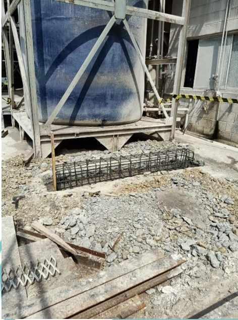
Lampiran 7: Foto pelaksanaan proyek instalasi progressive cavity pump
