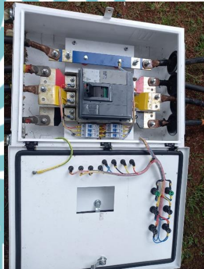
Gambar 3. 74 Panel Sinkron
