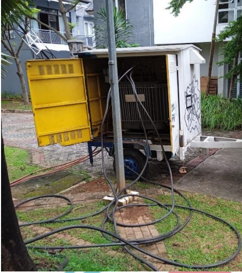
Gambar 3. 71 Unit Transformer Bergerak
