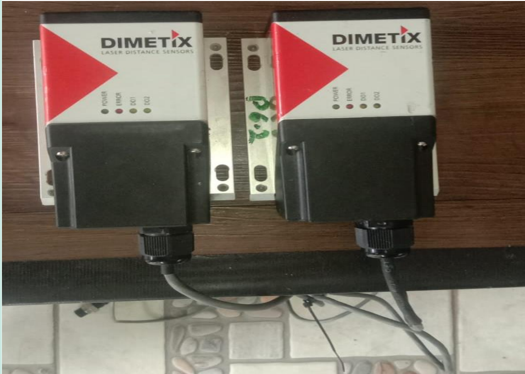
Foto 3. Sensor Laser Displacement
