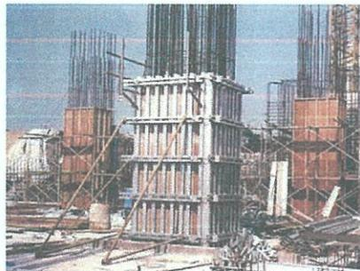
Gambar 19 . Bekisting Kolom
