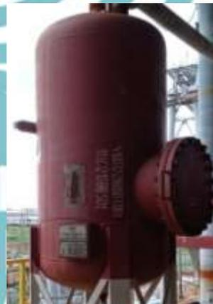
Gambar 3. 38. Continuous Blow Down Tank
