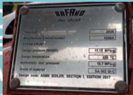
Gambar 3. 31.Name Plate of Steam Drum
