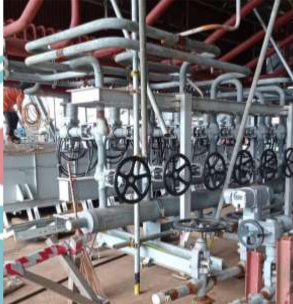
Gambar 3. 48. Line Drain and Manual Valve
