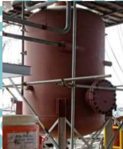
Gambar 3. 36. *Intermitten Blow Down Tank*
