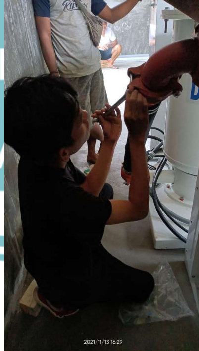
Proses penginstalasian Stabilizer dan pemasangan Interconnect Piping
