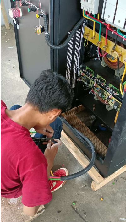
Proses penginstalasian Stabilizer dan pemasangan Interconnect Piping
