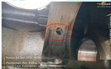
Condition actual Oil Jet Cylinder No.5 on seat (not fullyinstall)
