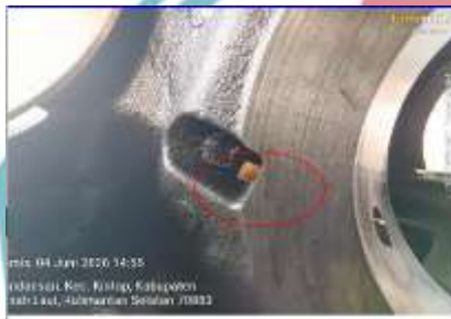
Condition actual Oil Jet Cylinder No.5 on seat (not fullyinstall)
