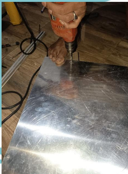
Lampiran 4 Proses Drilling Base Plate
