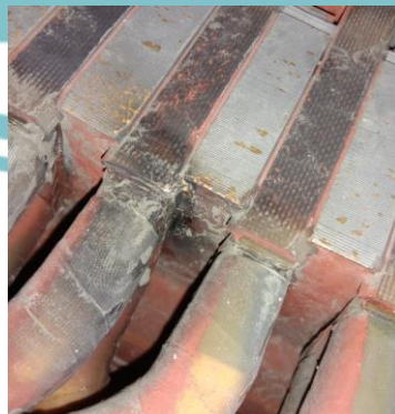
Gambar 4 7 Insulation Failure
