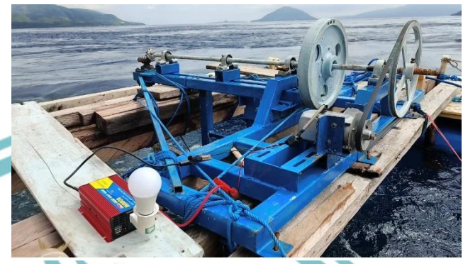
Fig. 2 (a) Installation of the MCPT on the pontoon, (b) The turbine in operation within the Pantar strait.
