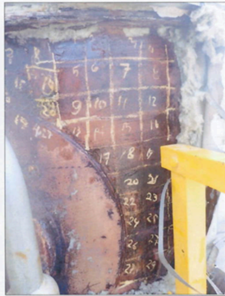
SHELL MH-2 AREA 2
