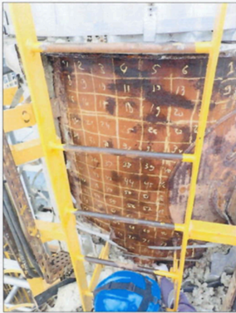
SHELL MH-2 AREA 3
