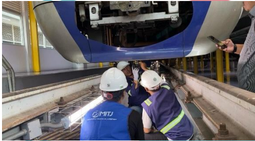
Documentation of the CBM Dismantling Project
