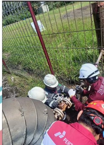
Memasang Steam trap
