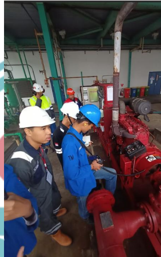
Pengambilan data vibrasi diesel fire pump
