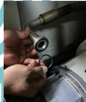
Penggantian O- ring Seal Hose
