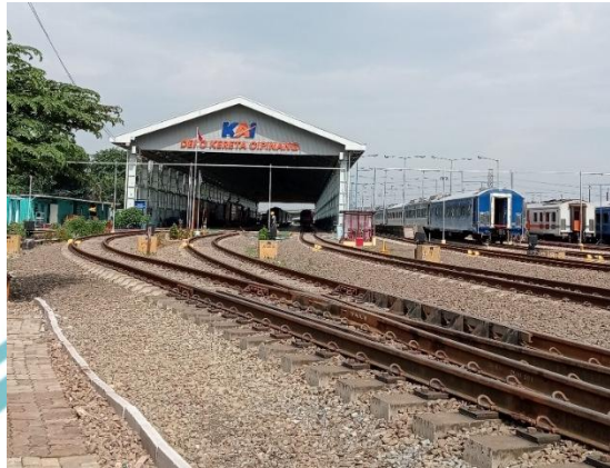
Gambar 1.2 Depo Kereta Cipinang
