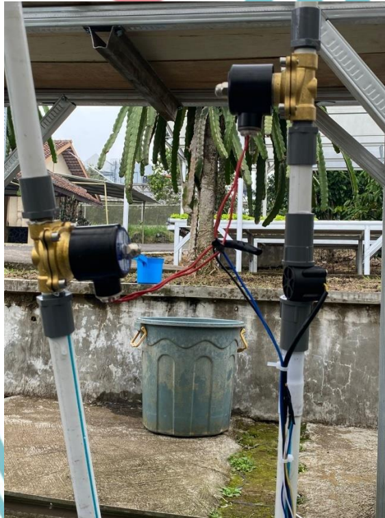
Gambar Realisasi Solenoid Valve & Flow Sensor
