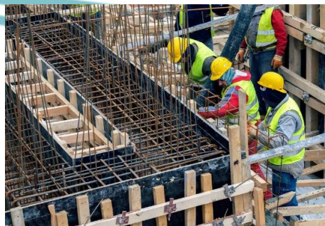
Gambar 2. 23 Bekisting Semi Sistem
