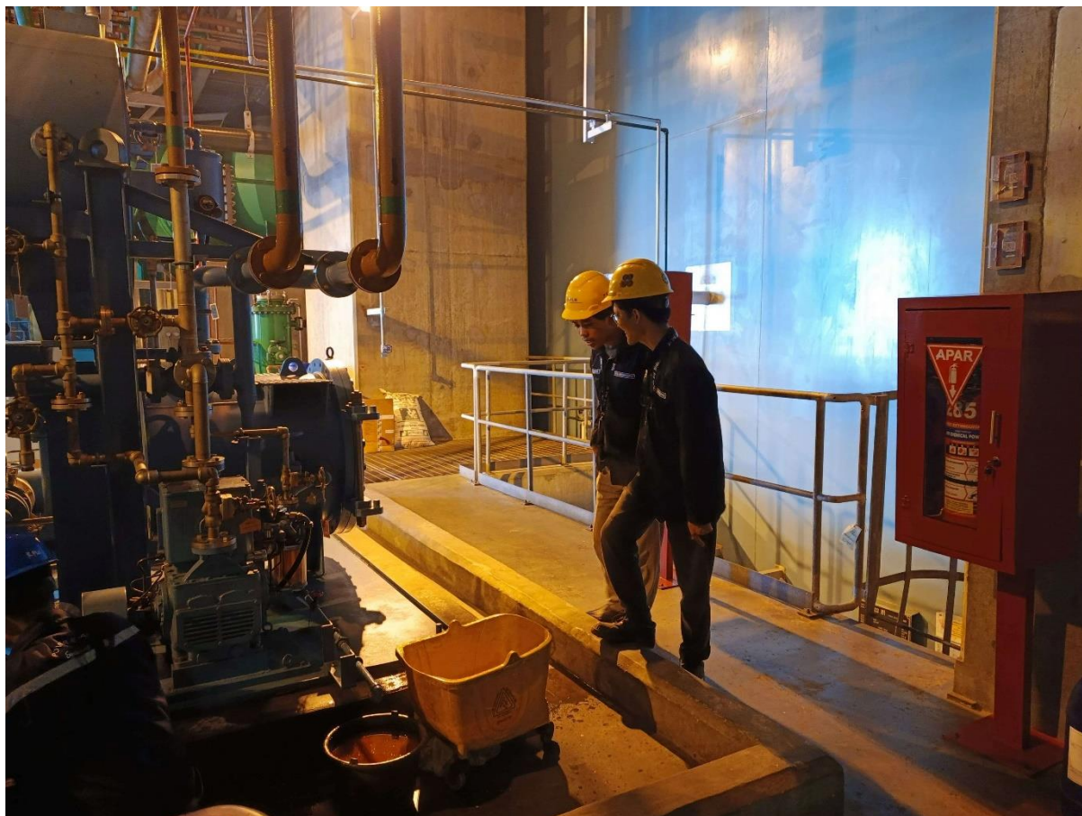
Lampiran 2.j Pengambilan data vibrasi main oil pump dan closed cooling water pump
