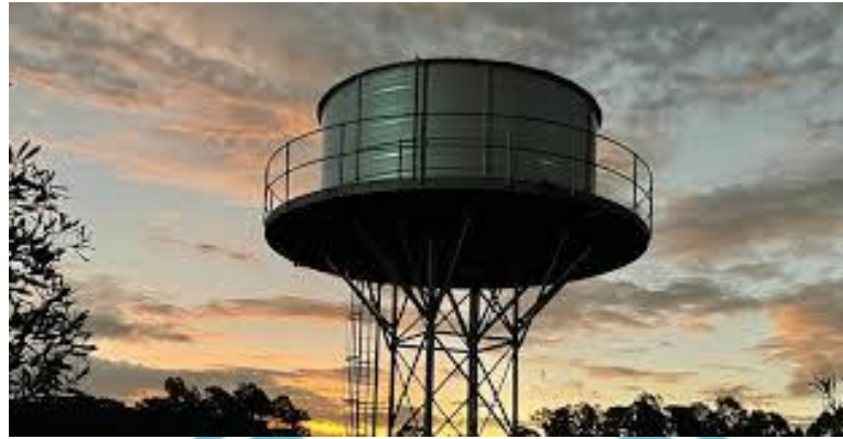
Gambar 2. 3 Elevated Reservoir Sumber : google image
