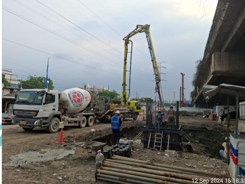
3.26 gambar pengecoran pilar stage 1
