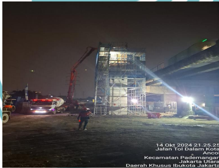
3.28 gambar pengecoran pilar stage 3
