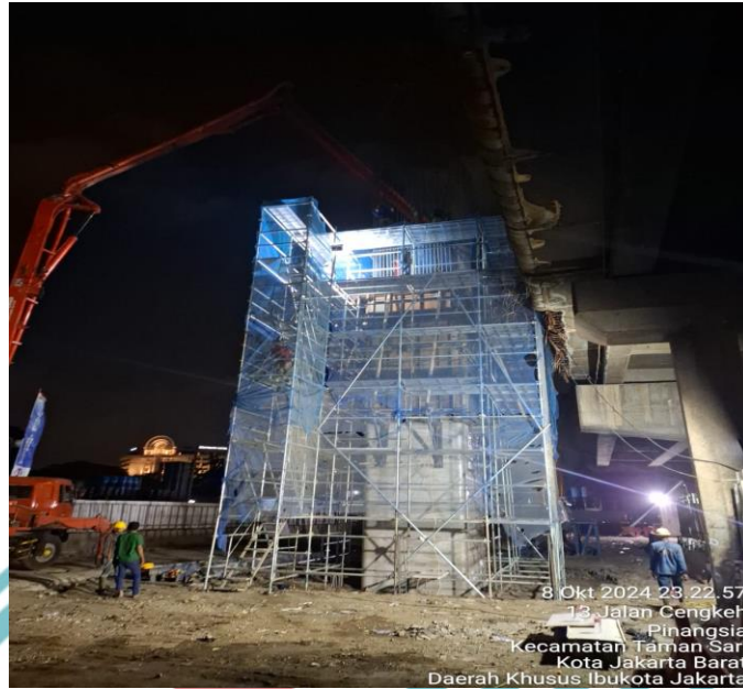
3.27 gambar pengecoran pilar stage 3
