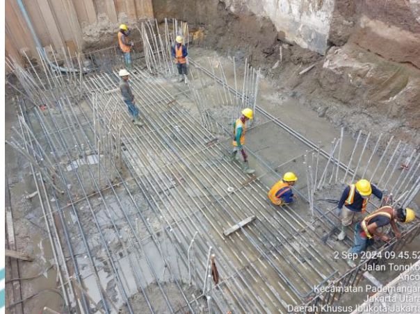
Gambar 3.16 cut off ujung bore pile
