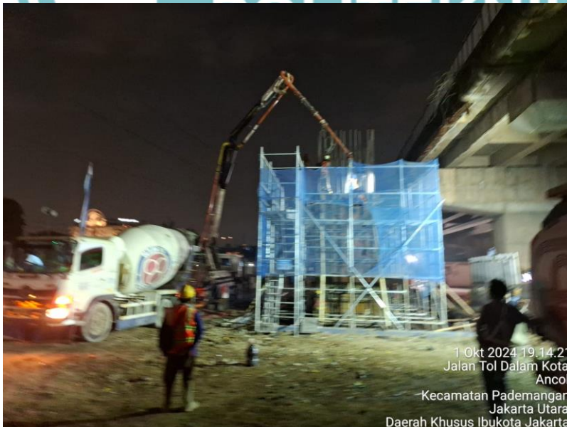
3.26 gambar pengecoran pilar stage 2
