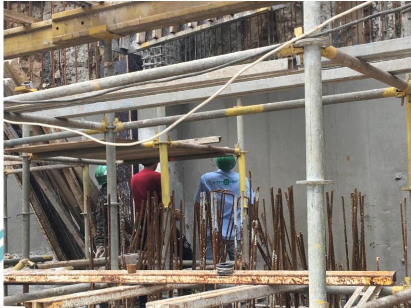
Gambar 3.19 Curing Beton Retaining Wall
