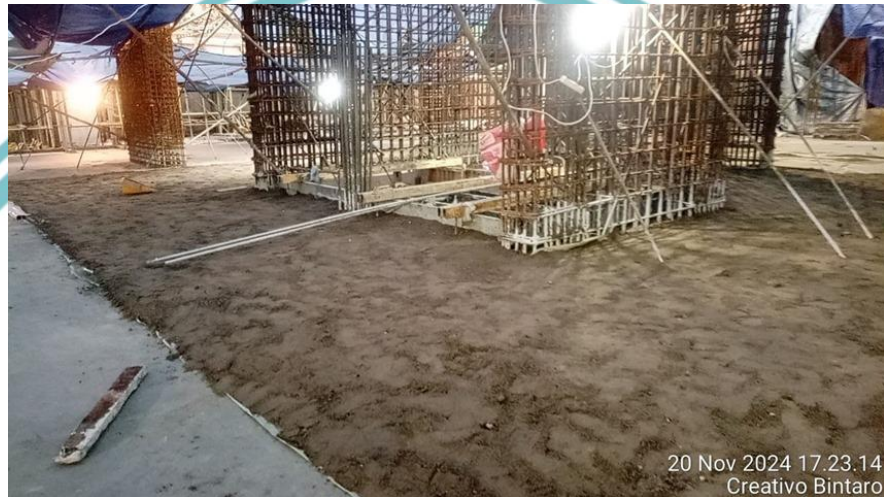
Gambar 3.42 Curing Beton Pondasi Raft
