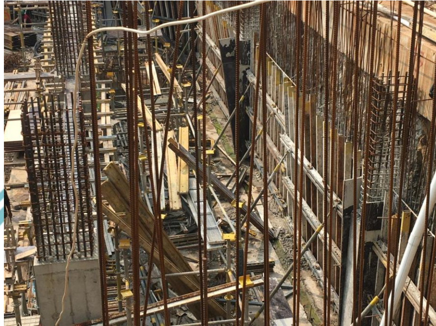
Gambar 3.17 Pekerjaan Bekisting Retaining Wall
