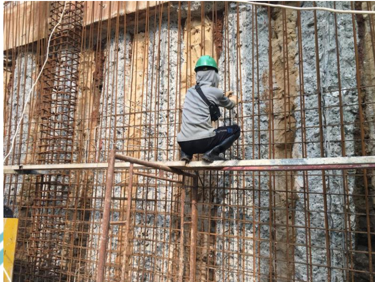
Gambar 3.16 Pekerjaan Pembesian Retaining Wall
