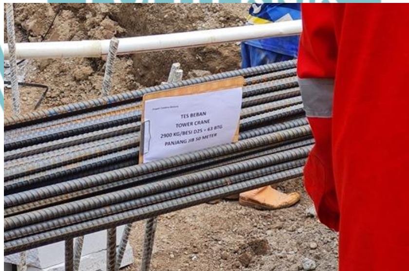
Gambar 3.57 Monitoring Pembebanan Tower Crane
