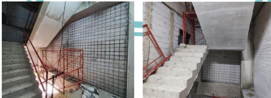
Gambar 3. 40 Monitoring Dinding Confinement
