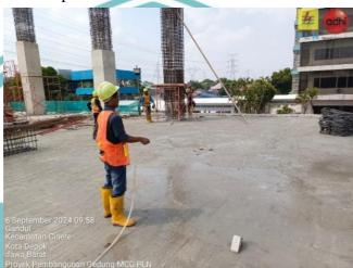
Gambar 3. 26 Curing Beton
