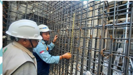
Gambar 3. 21 Checklist Struktur Retaining Wall
