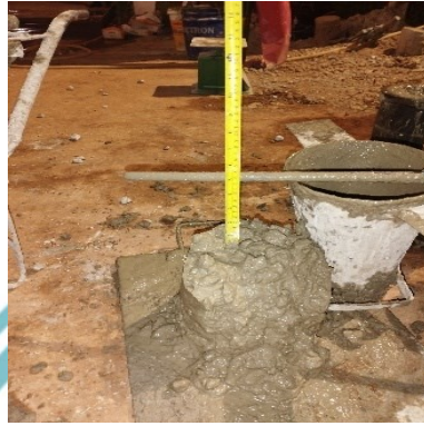
(Cek nilai slump )
