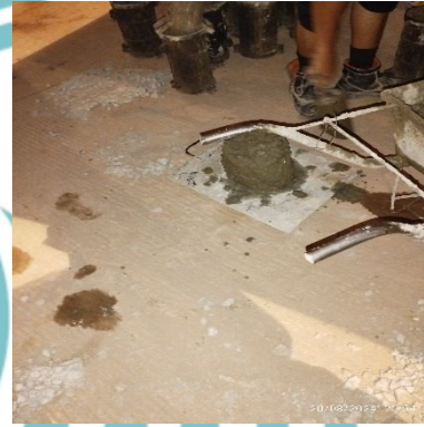
(Cek nilai slump )
