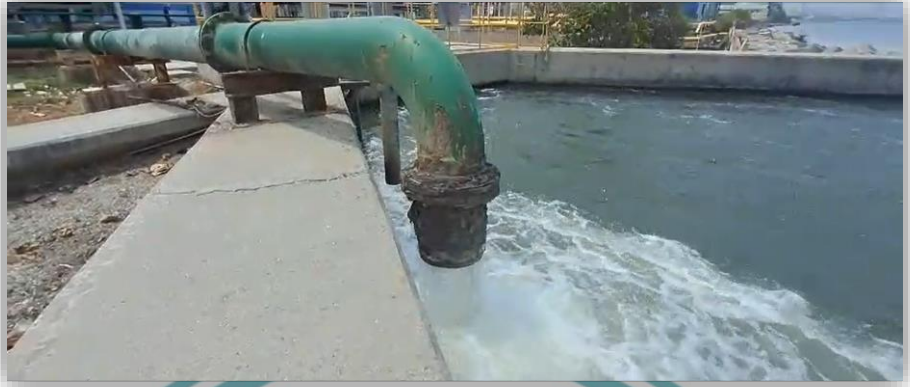
Gambar 1.1 Brine Blowdown Output Line
