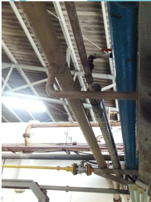
Sumber: Dokumen PT. GS BATTERY.
