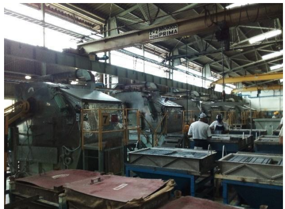
Sumber: Dokumen PT. GS BATTERY.
