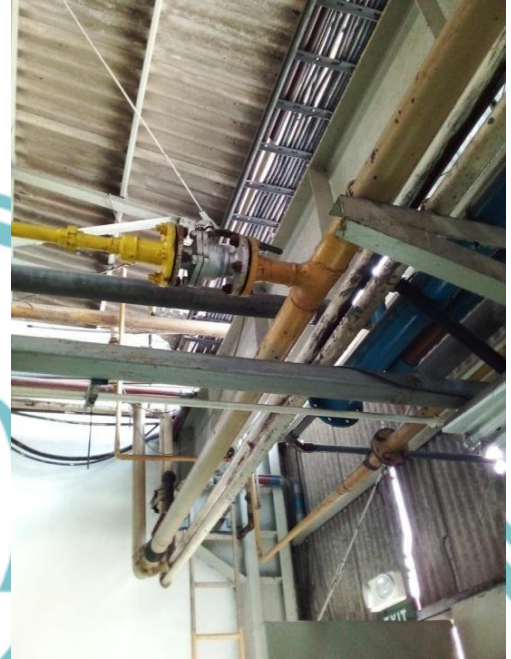
Sumber: Dokumen PT. GS BATTERY.
