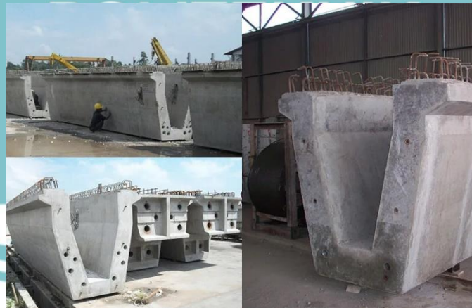
Gambar 2.3. 4 Girder Tipe PC-U
