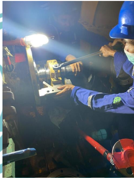
Proses Cek Clearance Journal Bearing
