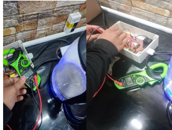
Fig 27 Testing Water Heater Using an Avometer
