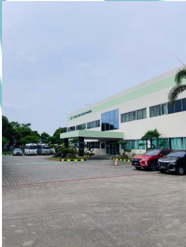
PT United Steel Center Indonesia (USC) Cibitung Plant
