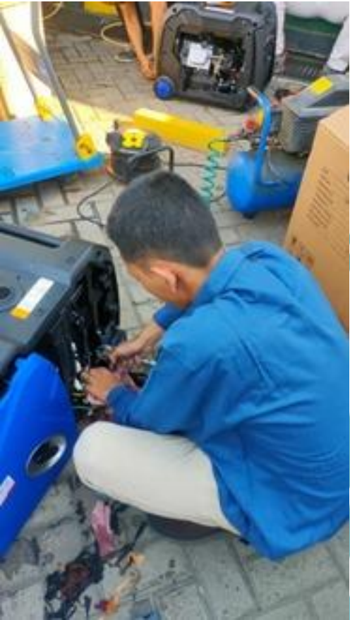
Test performance genset
