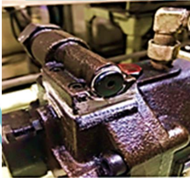
Lampiran 2 Aktifitas after re-sealing pada bagian bolt pressure
