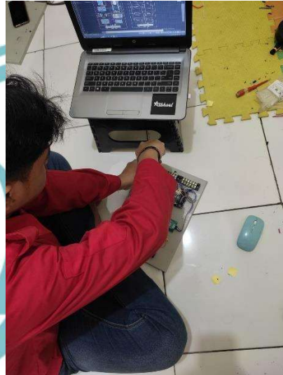
Proses Wiring Panel Kontrol
