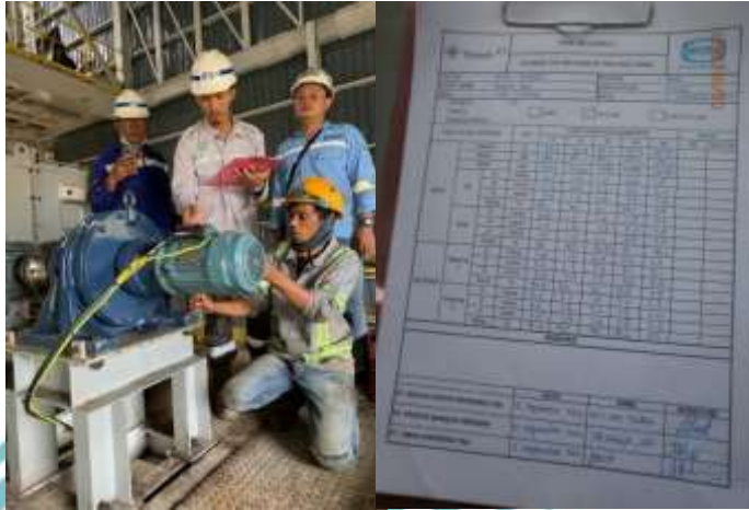
Mechanical Run Test
