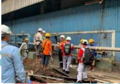
Inspeksi Tie -in Pipa
