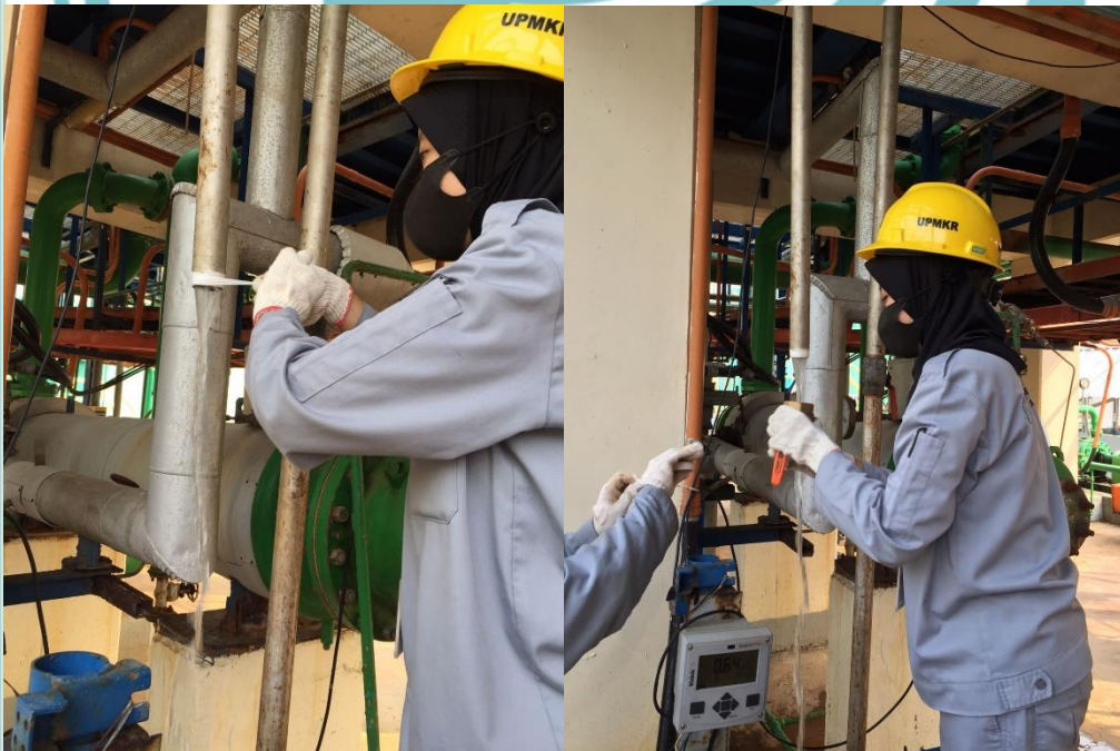
Gambar 8 Preventive Maintenance - Pemasangan Valve Draine Modul Evaporator Desal B
