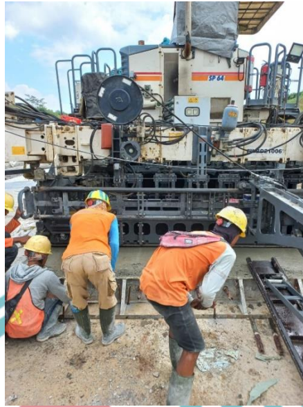
Gambar 4. 38 Pengecoran Rigid Pavement
