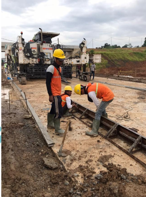
Gambar 4. 37 Persiapan Concrete Paver
