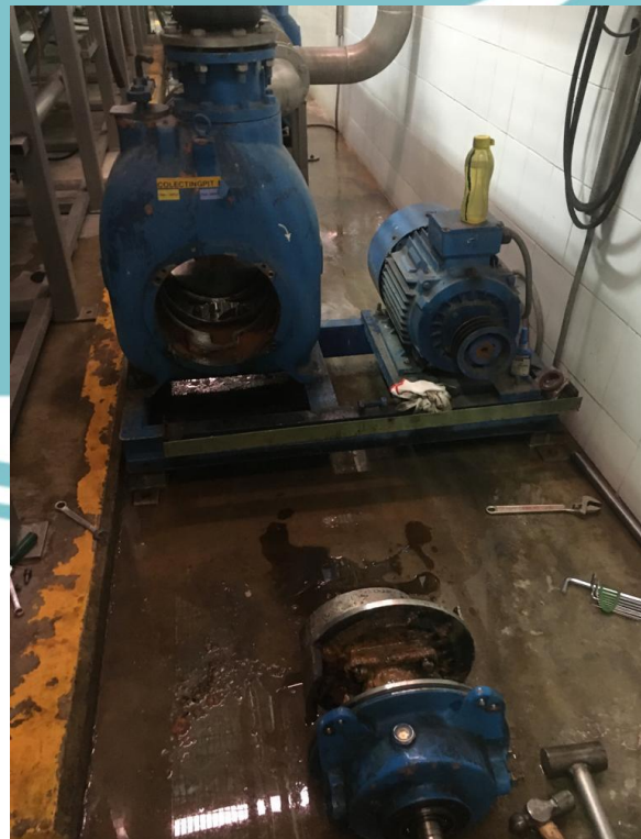
Membantu Mekanik Utility Mengganti Bearing Colectingpit Pump
