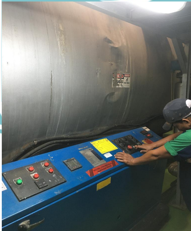
Membantu Operator Utility Menyalakan Boiler
