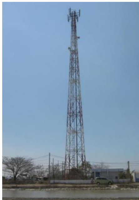
Gambar 2. 6 Tower Diatas Tanah
