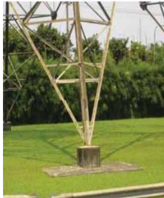
Gambar 2. 7 Pondasi Tower SUTET (Joko, Buwono, & Zamrudi, 2010)
