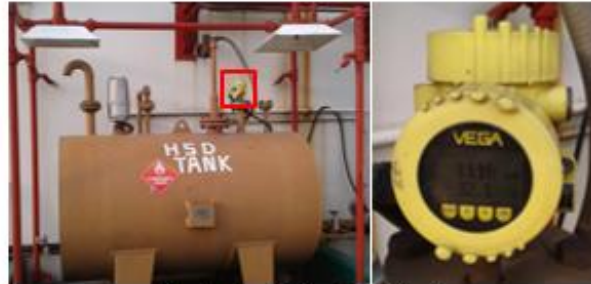
Gambar Level indicator HSD Tank
