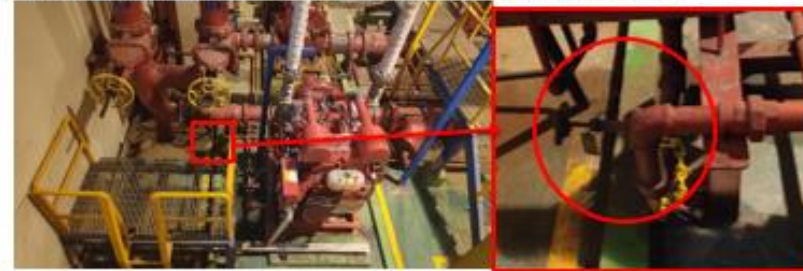
Gambar Isolation Valve pendingin diesel fire fighting pump
