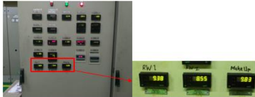
Gambar indicator level Raw Tank
