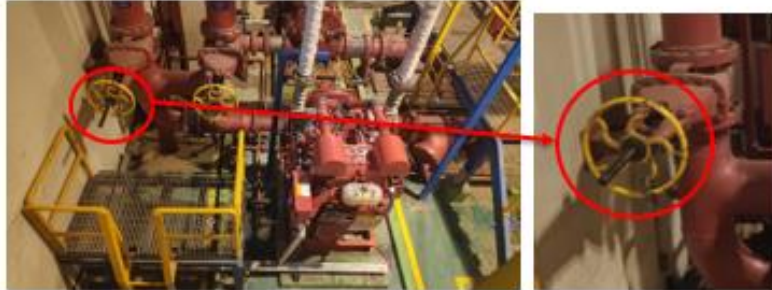
Gambar manual valve discharge to line 9oSGA01oAA0o4
