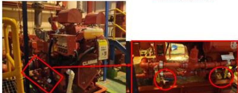
Gambar Isolation Valve pendingin diesel fire fighting pump
