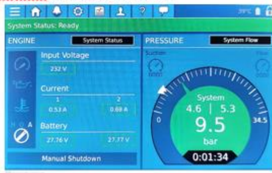
Gambar 2 Keterangan panel DC Engine Diesel Fire Pump
