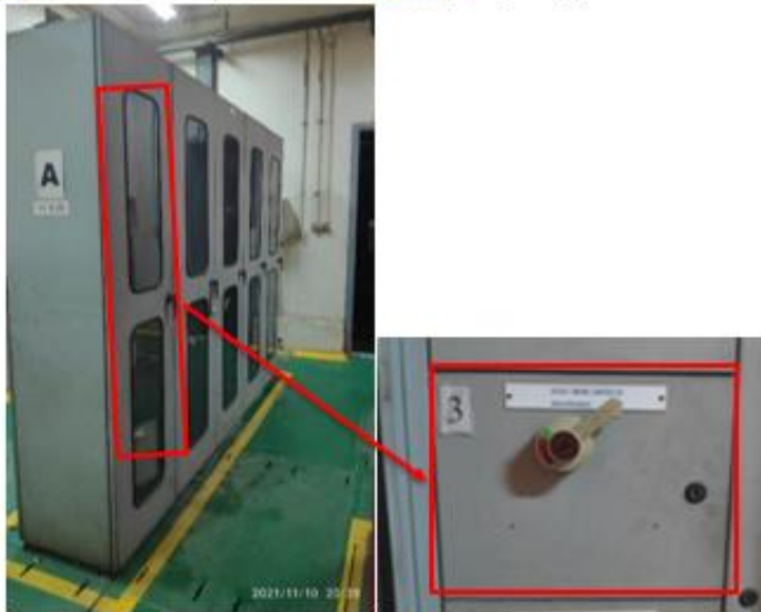
Gambar Breaker Diesel Engine Controller
