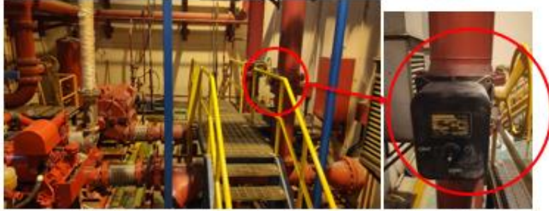
Gambar valve suction fresh water (raw water) 90SGA010AA004
