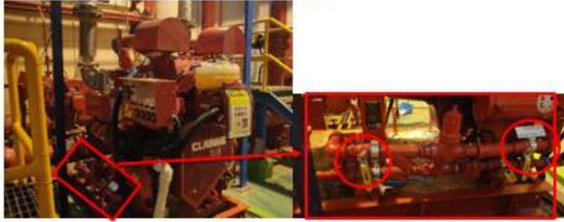
Gambar manual Valve by pass pendingin
