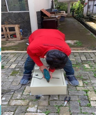
Lampiran 1. 1 Proses Melubangi Pintu Panel
