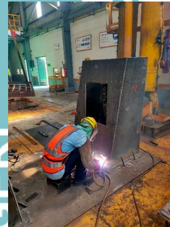
Proses Welding Chute
