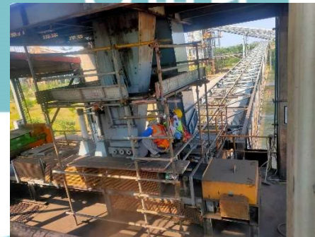
Proses Pra Instalasi
