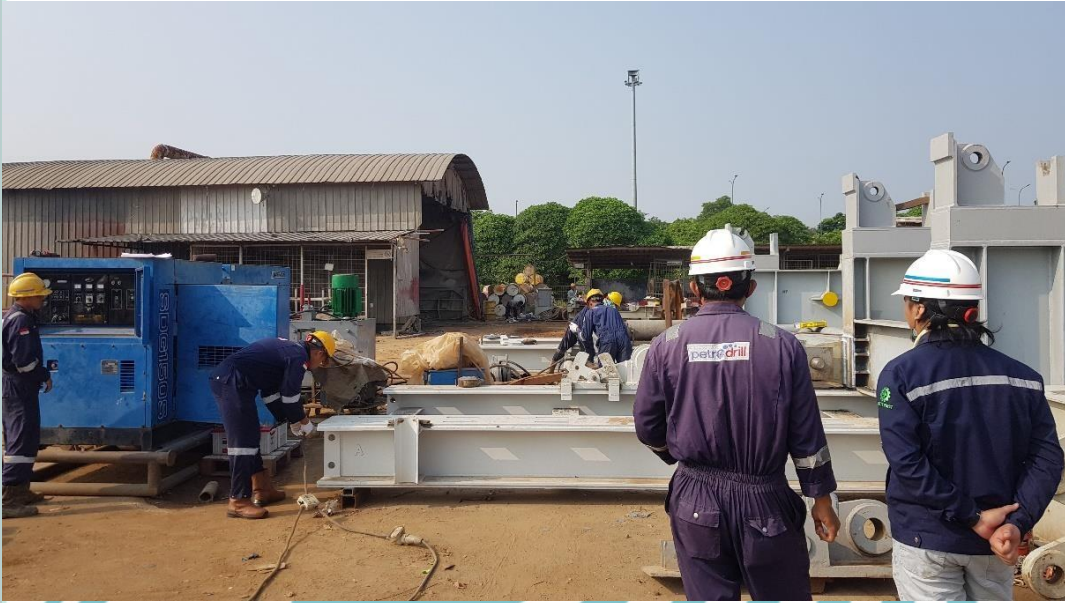
Proses skidding rel mast rig 550 hp
