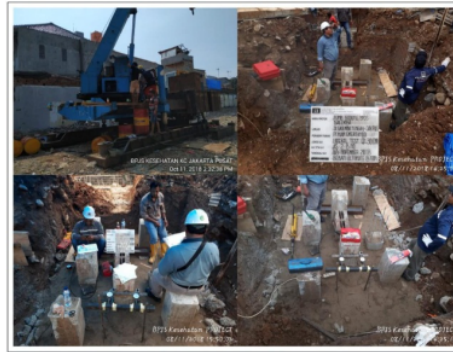
Figure 2: Piling and instalation of PDA test.
