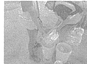
Mix SikaGrout 215 with Water
