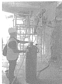
Use the pressure Grout to inject SikaGrout 215
