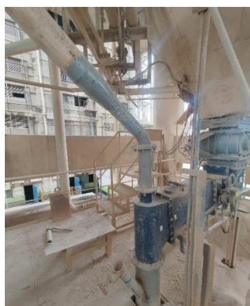
Gambar 2 Air Slide 4D2 – AS1
