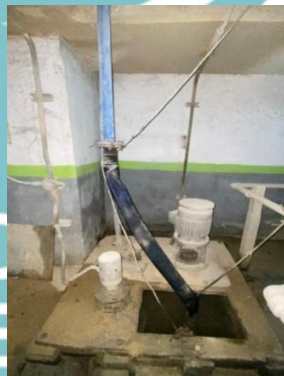
Gambar 1. 1 Area Underground Building Crusher
