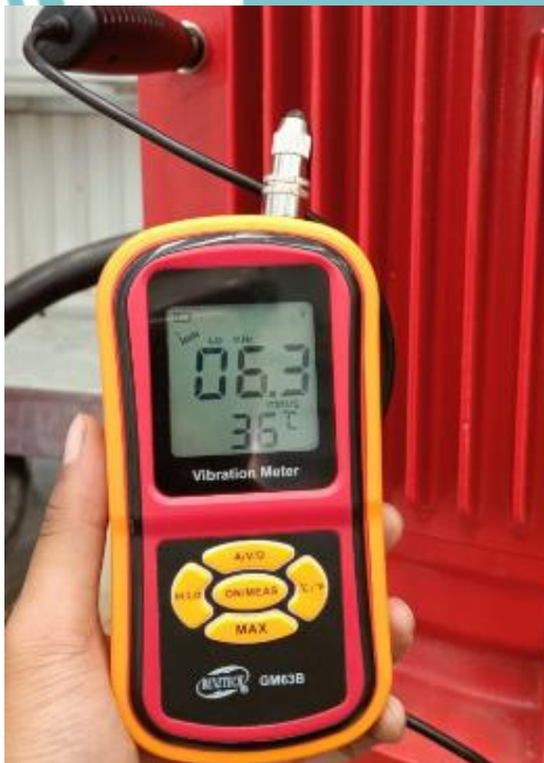
Inspeksi Getaran Water Pump
